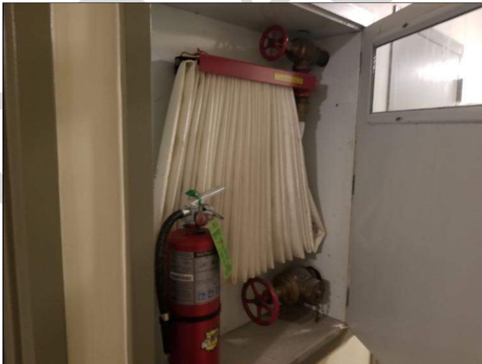
TYPICAL FLOOR STANDPIPE SYSTEM.
