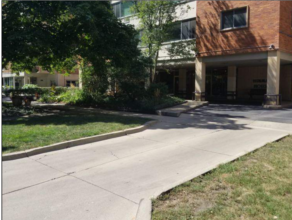
CLOSE-UP VIEW OF THE FRONT ENTRANCE (EAST ELEVATION) OF THE SUBJECT PROPERTY.
