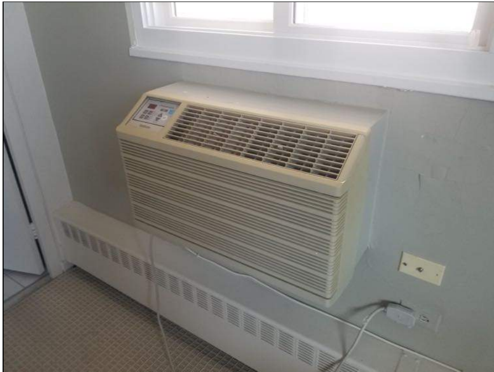
TYPICAL UNIT WALL A/C AND RADIATOR
