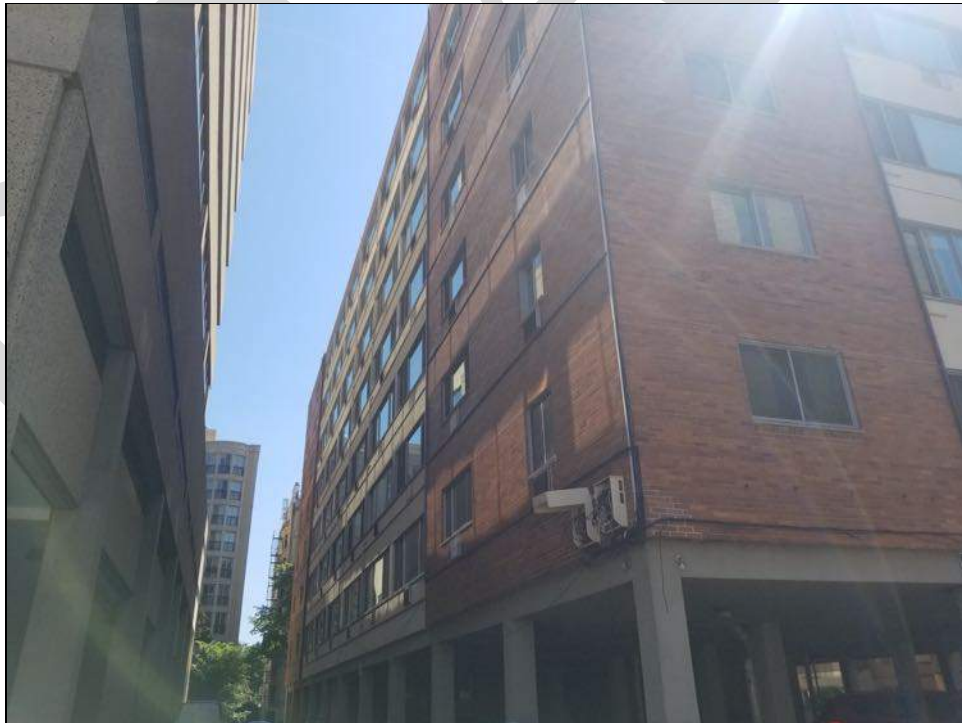
VIEW OF THE SIDE (NORTH ELEVATION) OF THE SUBJECT PROPERTY
