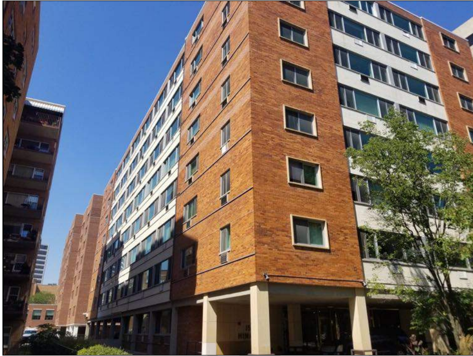
VIEW OF THE SIDE (SOUTH ELEVATION) OF THE SUBJECT PROPERTY
