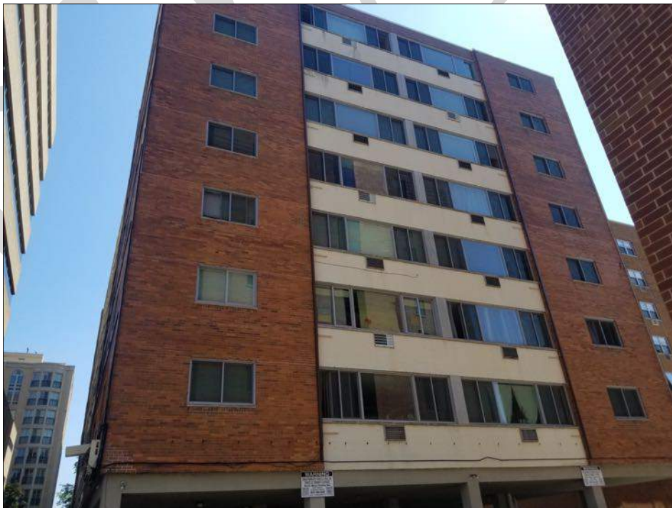
VIEW OF THE REAR (WEST ELEVATION) OF THE SUBJECT PROPERTY
