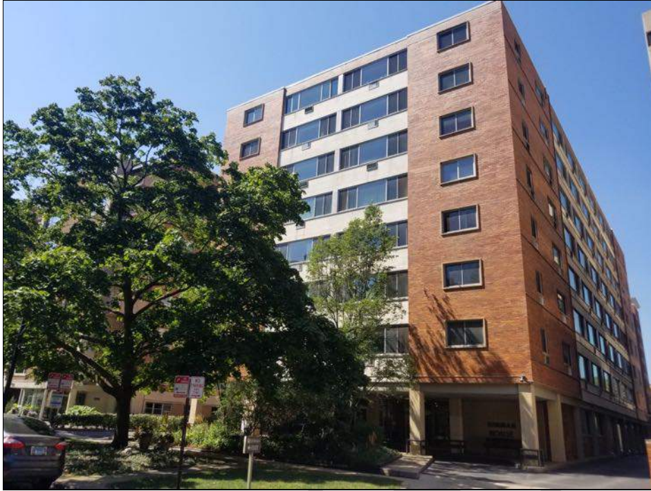
VIEW OF THE FRONT (EAST ELEVATION) OF THE SUBJECT PROPERTY
