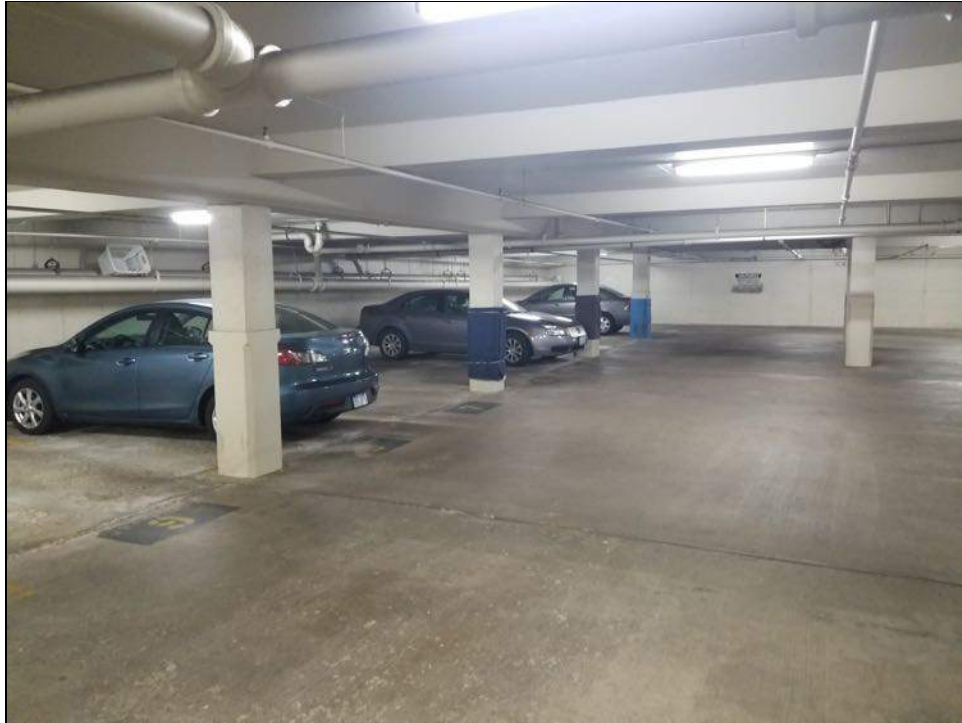
VIEW OF THE LOWER LEVEL GARAGE
