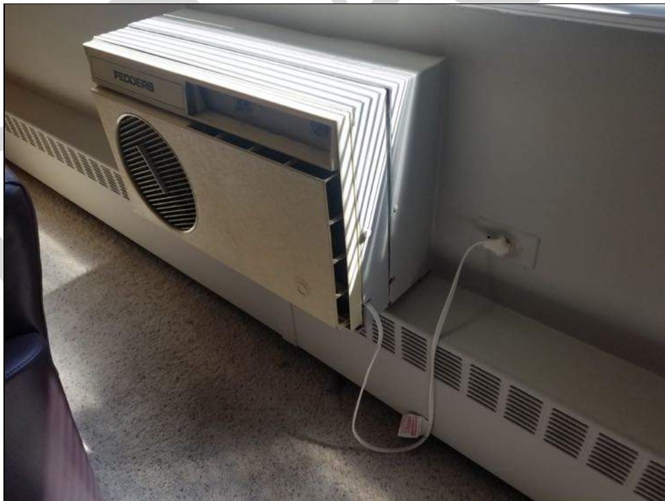
TYPICAL UNIT WALL A/C AND RADIATOR.
