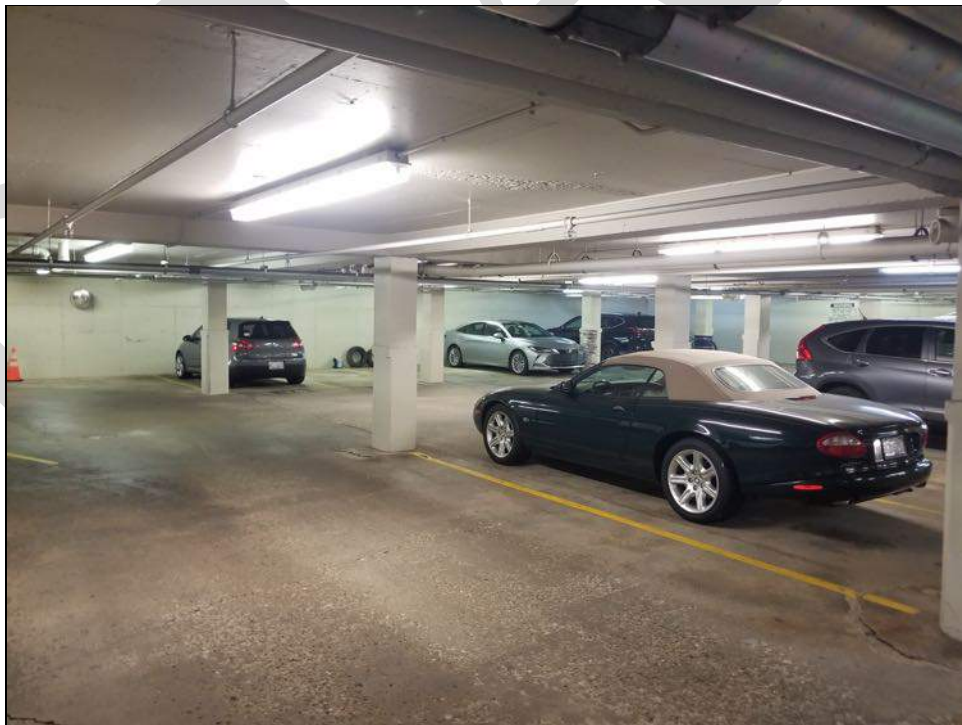
VIEW OF THE LOWER LEVEL GARAGE
