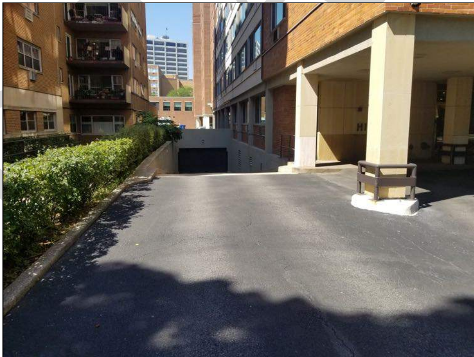
VIEW OF THE SOUTH SIDE ENTRY DRIVEWAY TO ENCLOSED GARAGE
