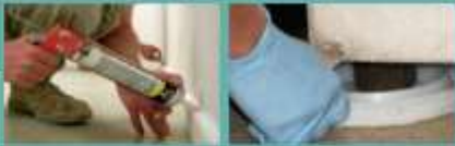
Caulk cracks and spaces Interceptor under leg
